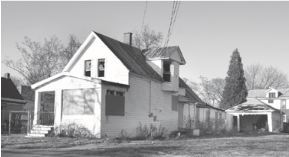
below: This abandoned house at 882 Northhanpton stands a block and a half away from East Comprehensive High School.
